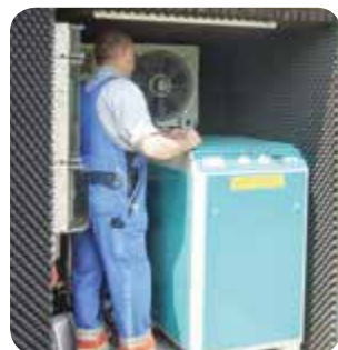
Concrete equipment cabinet
